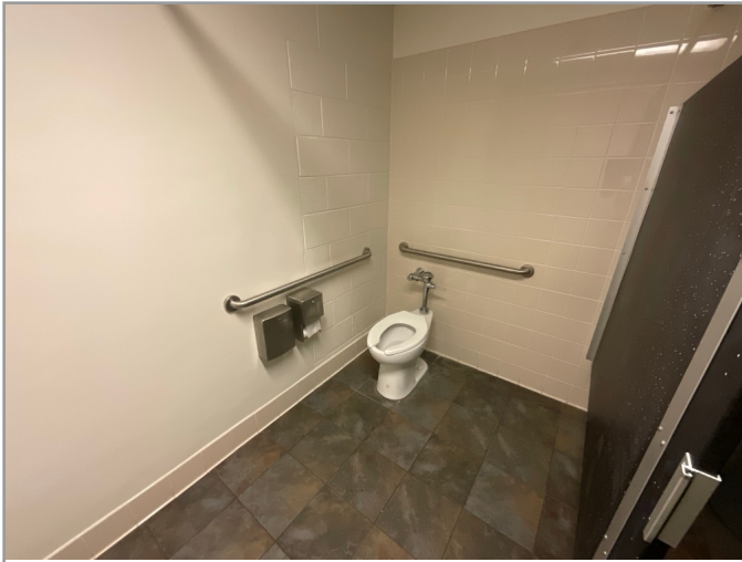
TOILET STALL OVERVIEW
