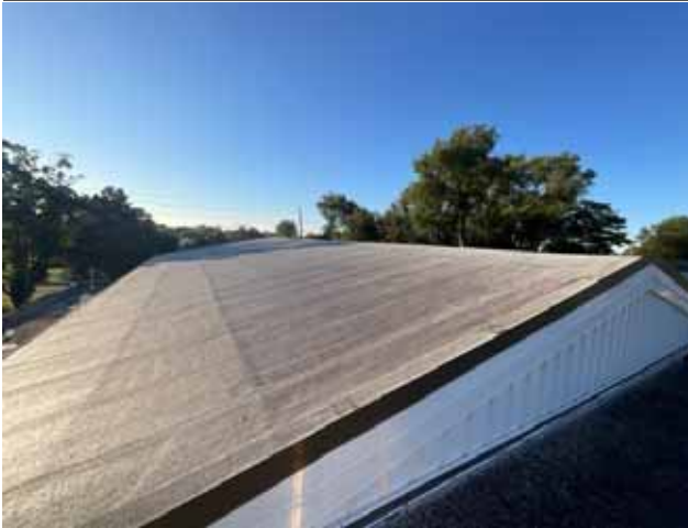
7 - GYMNASIUM ROOF OVERVIEW
