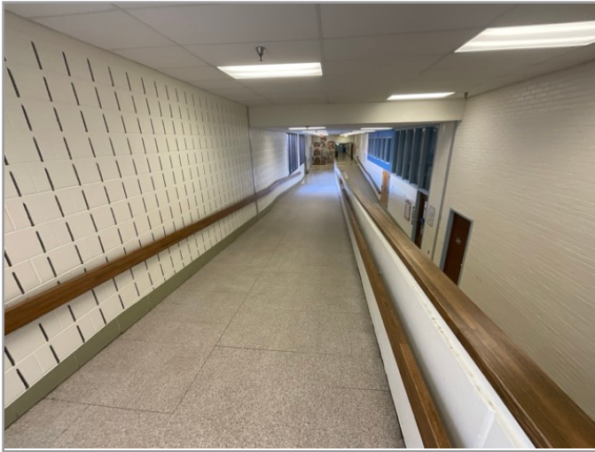
ACCESSIBLE INTERIOR RAMP
