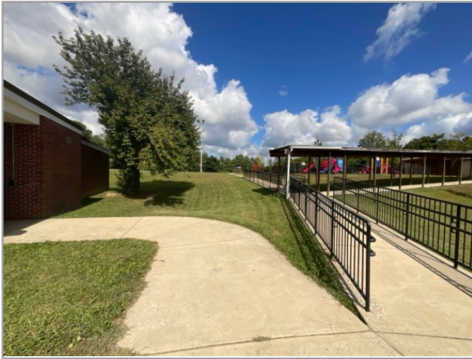
ACCESSIBLE ROUTE TO PLAYGROUND
