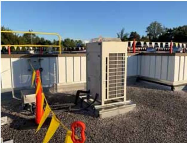
27 - HEAT PUMP VRV UNIT
