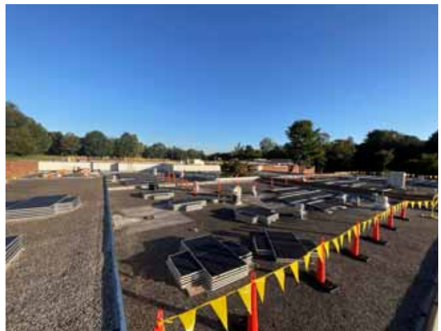
6 - MAIN ROOF OVERVIEW
